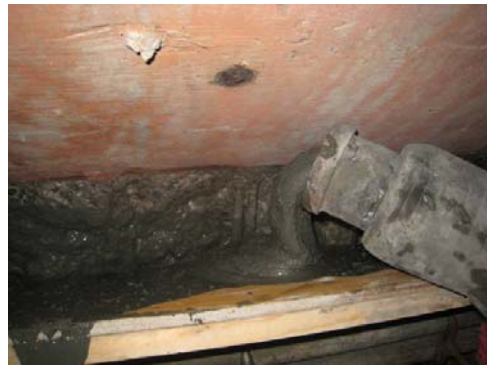
Photo 14 型枠へのポンプ圧送状況 Pumping to a form
