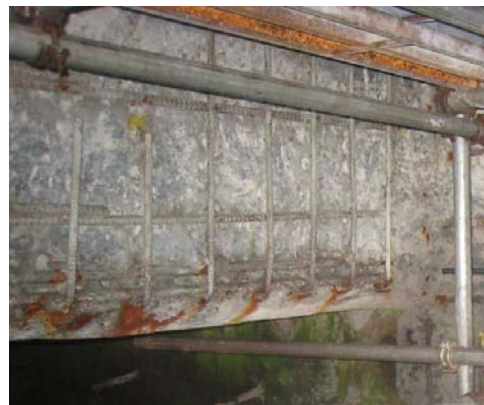
Photo 10 梁劣化部除去 Removal of the beam deterioration department
