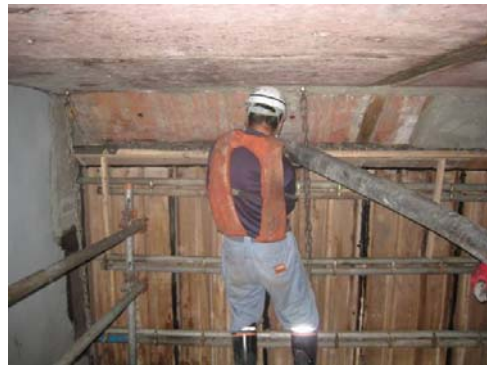
Photo 13 型枠への打設状況 Construction of the Slim Creat
