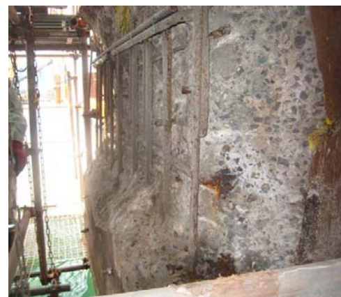
Photo 11 柱劣化部除去 Removal of the pillar deterioration department
