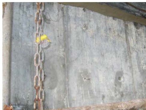
Photo 16 柱部仕上がり状況 Finish of the Slim Creat pillar
