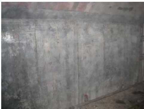
Photo 15 梁部仕上がり状況 Finish of the Slim Creat beam
