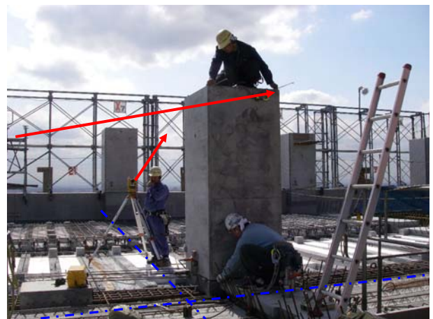
Fig. 10 PCa工事における在来測量 Conventional Surveying at Precast Concrete Construction
