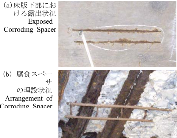
Photo 8 腐食スペーサの埋設状況 Arrangement of Corroding Spacer
