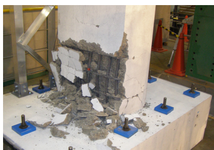
Photo 5 橋脚基部の損傷(ダンパーなし, L2) Damage of Pier (No-Damping, Level-2)
