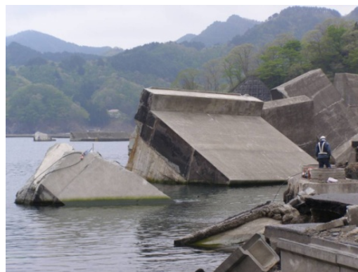
Photo 1 津波被害 Damage by Tsunami
