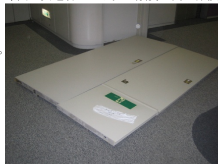
Photo 4 防火戸の被害事例 Damage of Fire Doors
