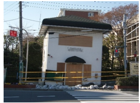
Photo 3 液状化被害 Liquefaction
