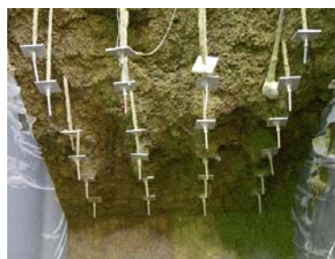
Photo 2 崩壊状況 (Case2-20mm) Slope Failure (Case2)
