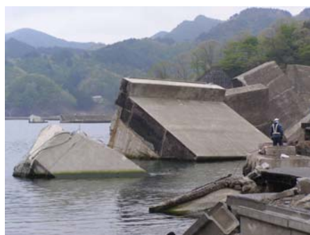
Photo 2 両石地区の防潮堤転倒 Overturning of Seawalls at Ryoishi Area
