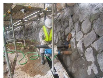
Photo 2 削孔状況 Construction Situation
