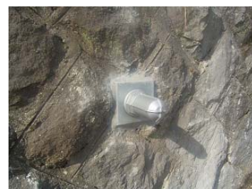
Photo 4 補強材頭部の状況 View of Nailing
