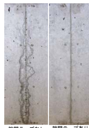
Photo 5 隙間テープによる砂すじの防止効果 Effect of the Airtight Tape on Reduction of Sand Streaking
