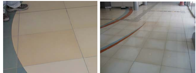
Photo 1 全面型黄変 Full-scale Type Yellowing
