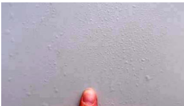
Photo 2 膨れの発生状況 Blister at the Coating
