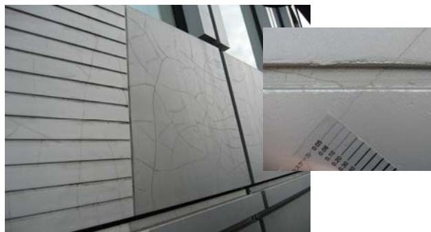
Photo 1 塗膜表面の微細なひび割れ Minute Crack at the Coating
