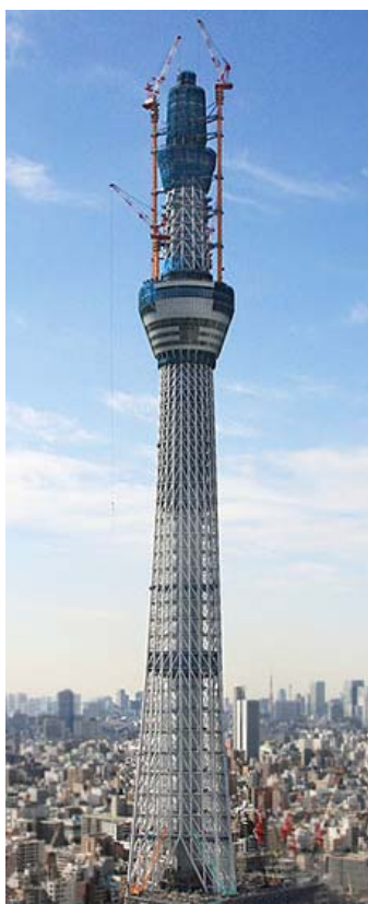
Fig. 1 塔体鉄骨工事の状況 A State of Steel Work of the Main Tower
