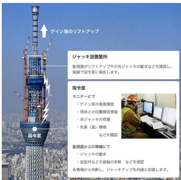
Fig. 7 リフトアップ工事指令室の概要 The Control Cabin in the Gain Tower Lifting-up Work
