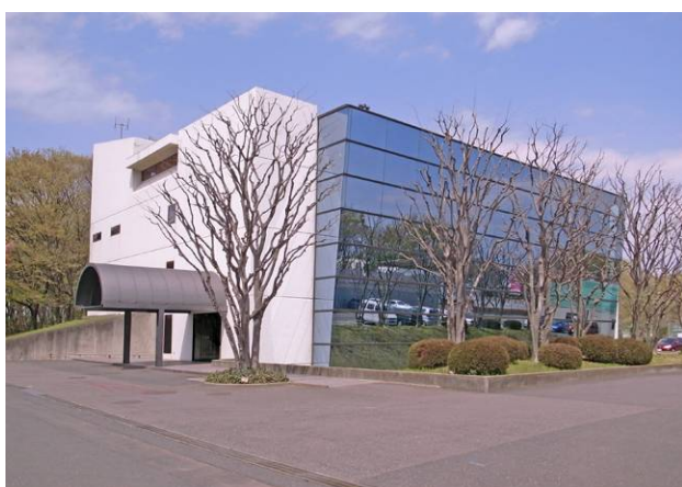
Photo 1 改修前全景 Existing Building
