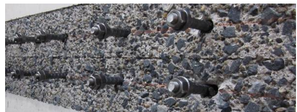
Photo 1 WJ目粗し状況 Condition of Concrete Joint with Roughness by Waterjet Technique
