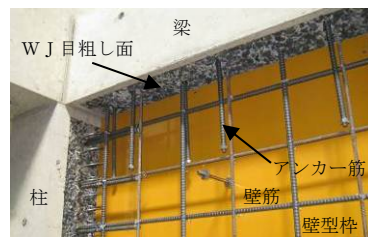
Photo 4 WJ目粗し状況 Condition of Concrete Joint with Roughness
