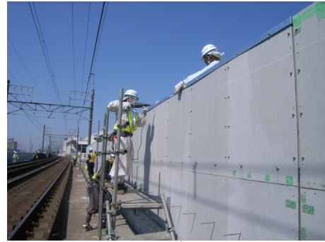
Photo 3 施工状況 Construction phase of this method
