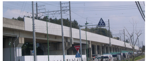
Photo 4 完成状況（左端は嵩上げ前） Parapet Wall after applying this method
