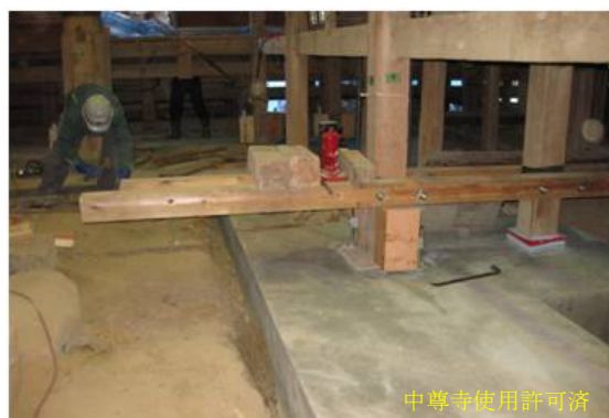
Photo 5 RC 基礎の施工 Reinforced Concrete Foundation
