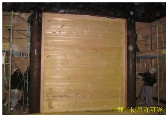
Photo 6 スーパー板壁設置状況 Installation of Super Wooden Wall
