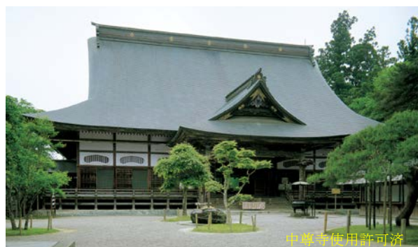
Photo 3 建物外観 Exterior of Chusonji-Temple Hondo
