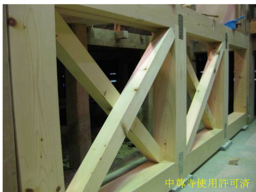
Photo 4 床の下の筋違補強 Reinforced Under Floor by Braces
