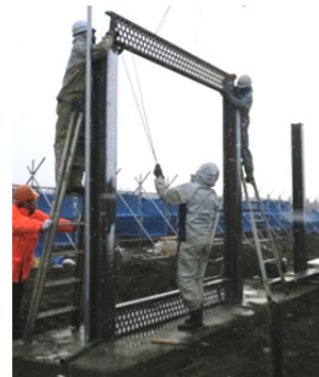
Photo 2 施工状況 Construction Situation
