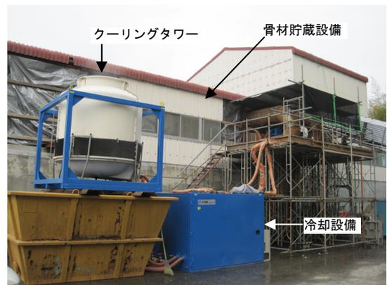
Photo 2 骨材の冷却設備 Cooling Equipment of Aggregate
