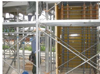
Photo 6 柱型枠の取付
