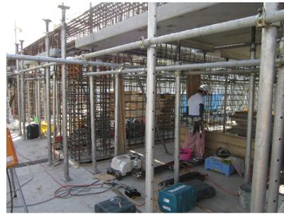
Photo 11 壁型枠の取付
