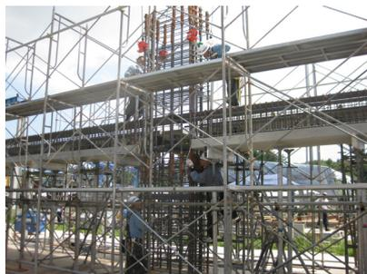
Photo 4 柱筋の取付
