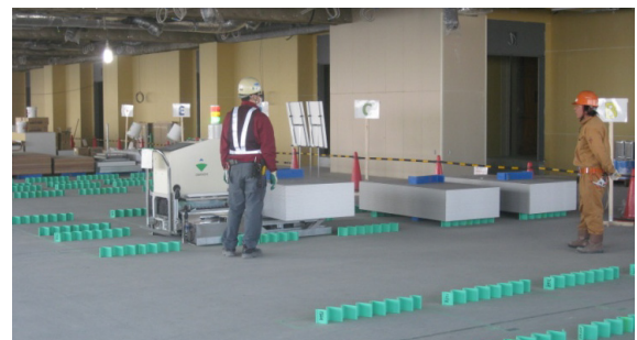
Photo 6 資材の仮置 Material Temporary Placement
