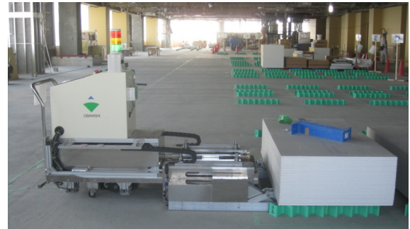
Photo 5 荷取位置での資材の積載 Loading Material at Pick-up Location
