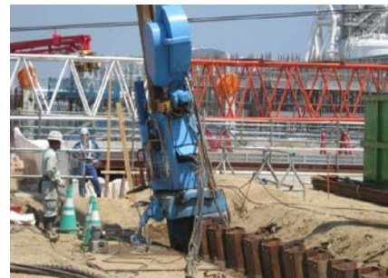
Photo 7 斜め土留め打設状況 Overall View of Driving Work
