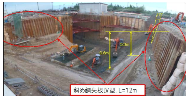
Photo 8 斜め土留め掘削完了状況 Overall View of Excavation Completed Site
