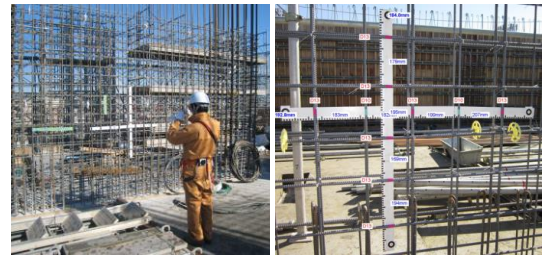
Photo 2 配筋自動判定システムの現場適用状況 Application of the Automated Bar Arrangement Checking System to Construction Sites
