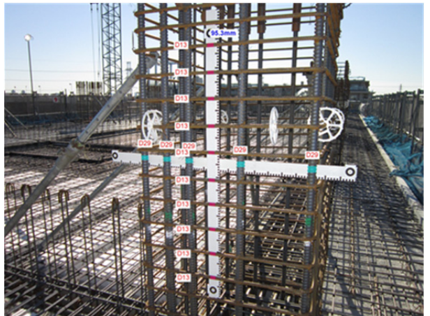
Photo 7 柱筋への適用 Application to Reinforcement of a Column
