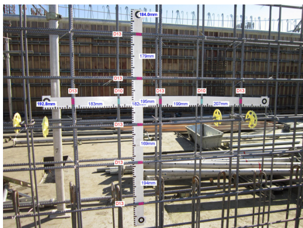
Photo 8 壁筋への適用 Application to Reinforcing Bars of a Wall
