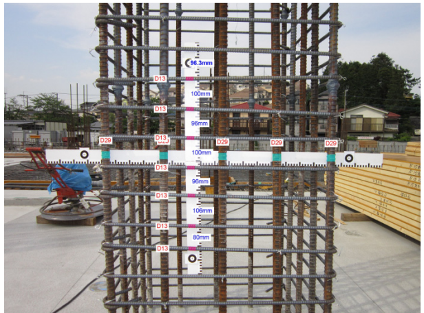
Photo 6 柱筋への適用 Application to Reinforcement of a Column
