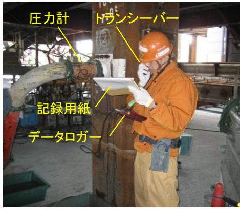
Photo1 従来の圧力管理方法 Conventional Pressure Measurement Method
