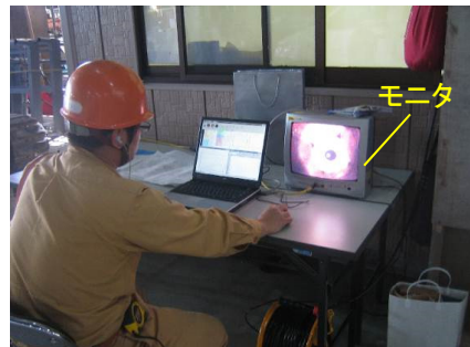
Photo7 管内カメラによる高さ記録 Placing Height Measurement by Image of Cable Camera
