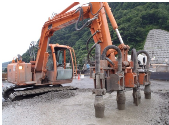
Photo 3 締固め判定現場試験状況 The Field Test Situation
