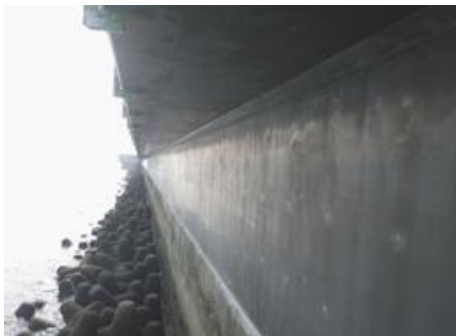
Photo 10 脱型状況 The Completion of Renewal
