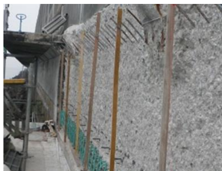
Photo 7 既設構造物の撤去状況 After Removal of a Degradation Part
