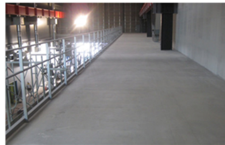
Photo 4 スラブの状況 Slab of Low Drying Shrinkage Concrete
