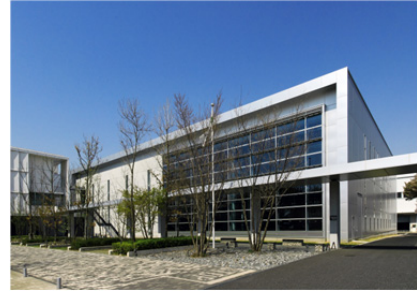
Photo 1 建物の外観 Appearance of New Laboratory
