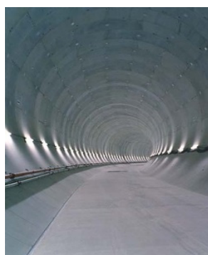
Photo 5 首都圏外郭放水路 The Metropolitan Area Outer Underground Discharge Channel
