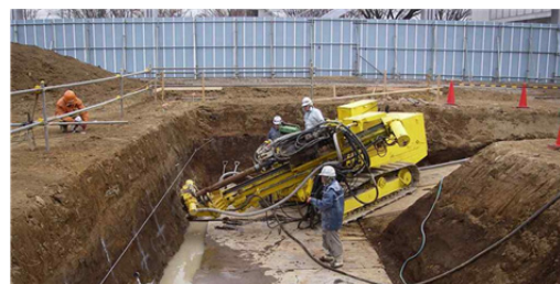
Photo 6 試験施工状況 View of Executing of High Spec Nailing
