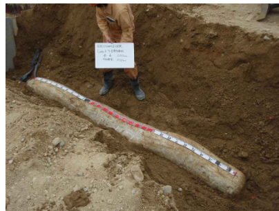
Photo 5 出来形確認 View of the Specimen after Test
