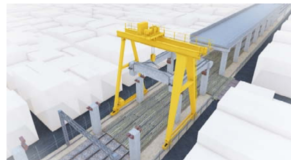
Fig. 14 鉄道高架橋へのLRV工法の適用 Application of "LRV" Method to the Railway Viaduct
