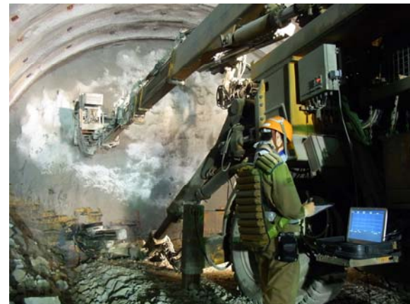
Photo 5 ノンコア削孔探査技術トンネルナビ Non-core Drilling Exploration System "Tunnel Navi"
