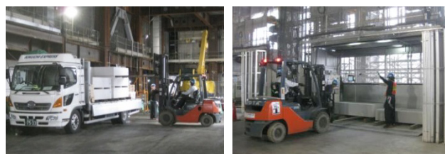
Photo 10 搬入状況 Carrying Materials into site
