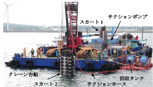
Photo 1 貫入実験状況 Field Penetration Tests
