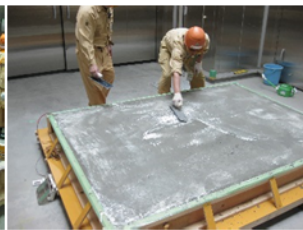
Photo 6 養生剤塗布状況 Applying the Curing Agent
