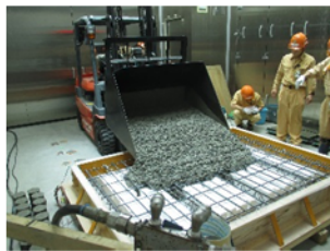
Photo 5 打込み状況 Concrete Placement
