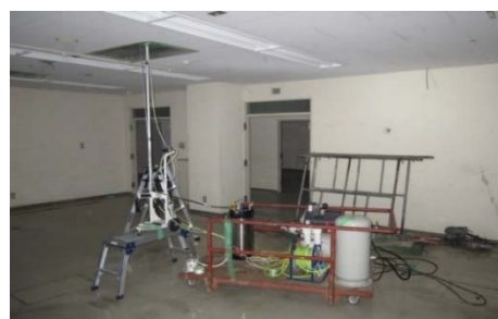
Photo 4 天井裏除カビ工事 Construction Work of Decontamination of Fungi
