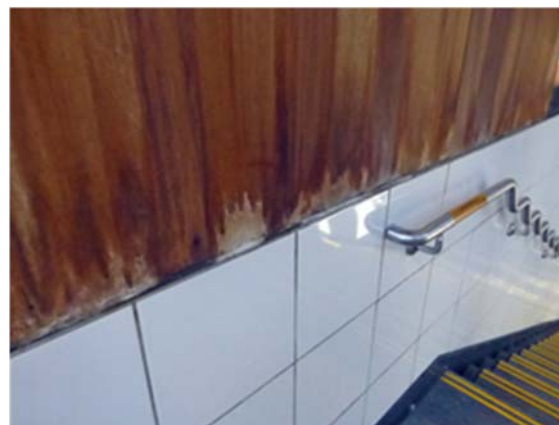
Photo 1 不燃木材表面の白華 Efflorescence of Incombustible Lumber
