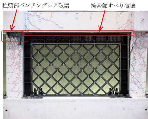
Photo 5 試験体Jgs2の最終破壊状況 Failure State of Specimen Jgs2
