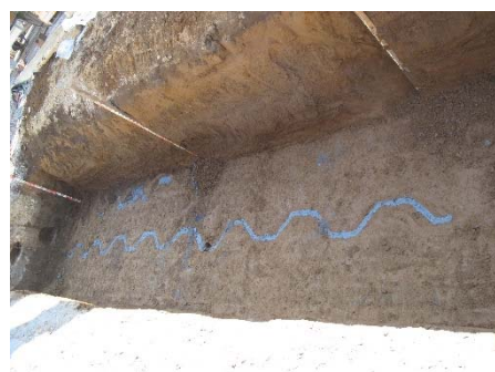
Photo 6 遮水壁の厚さ分布 Distribution of Thickness of Water Barrier Wall
