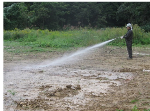
Photo 4 PIC 散布状況 Spraying of Polyion Complex Solution
