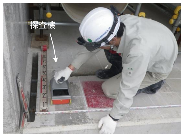
Photo 11 鉄筋探査の状況 Rebar Investigation using a Radar
