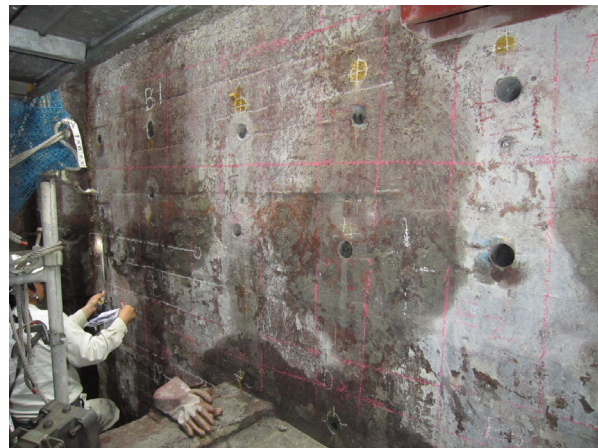
Photo 2 削孔状況 Drilled Holes at the Wall
