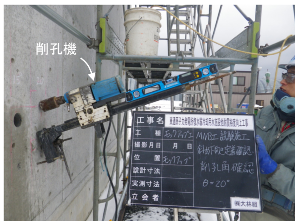
Photo 8 斜め下向き施工における削孔機セット状況 Side View of Core-Drill Set at Downward Slope
