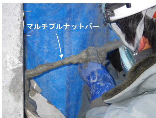
Photo 9 斜め下向き施工におけるグラウト状況 Multiple-Nuts-bar Insertion in case of Downward Slope
