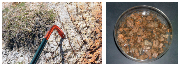
Photo 10 試料採取と測定時の水浸状況 Sampling and Dipping State of Chipcrete
