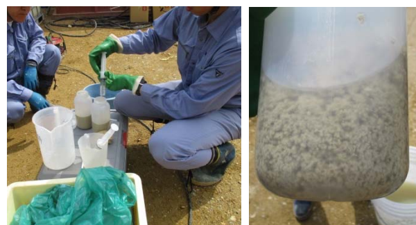
Photo 1 現場予備試験状況 Situation of sample test
