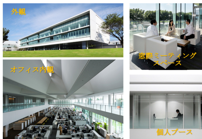
Photo 1 本館の外観および内観 External and Internal Appearance of Main Building
