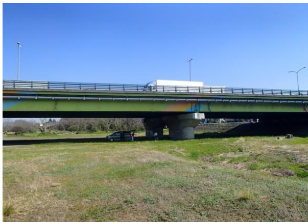
Photo 2 計測対象の橋梁 Measured Bridge
