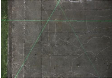
Photo 9 ひび割れ検出面1 Example of Concrete Surface 1
