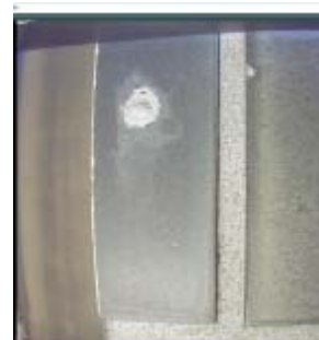
補修跡 Remains of Repair
