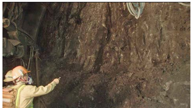
Photo 1 切羽観察状況 Observation of Tunnel Face
