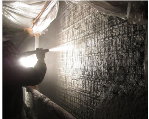
Photo 3 吹付けの状況(壁面) Situation of Shotcrete (Wall)
