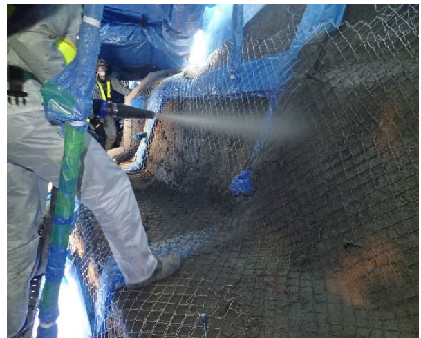
Photo 4 吹付けの状況(のり面) Situation of Shotcrete (Slope Protection)
