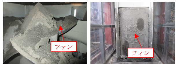
Photo 5 空調室外機に付着した火山灰 Volcanic Ash Attached to Air Conditioning Equipment
