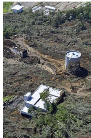
Photo 2 胆振東部地震による土砂崩れで壊滅的な被害を受けた富里浄水場(北海道厚真町, 読売新聞社撮影) Tomisato Water Purification Plant; Damaged by Large-scale Landslides Caused by the Iburu Eastern Earthquake
