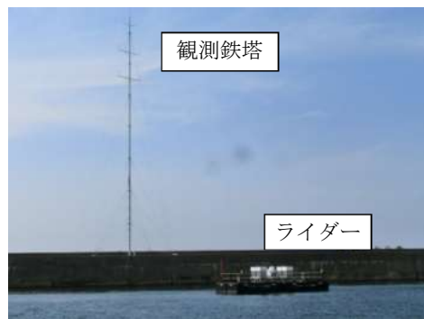
Photo 2 観測状況 (能代港) Situation of Observation
