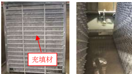
Photo 3 冷却塔に付着した火山灰 Volcanic Ash Attached to Cooling Tower
